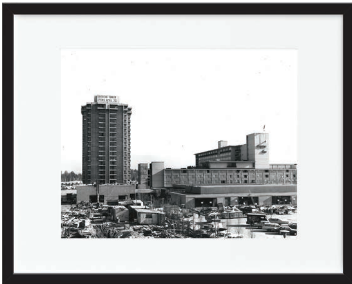
Tower Construction - March 3, 1970
